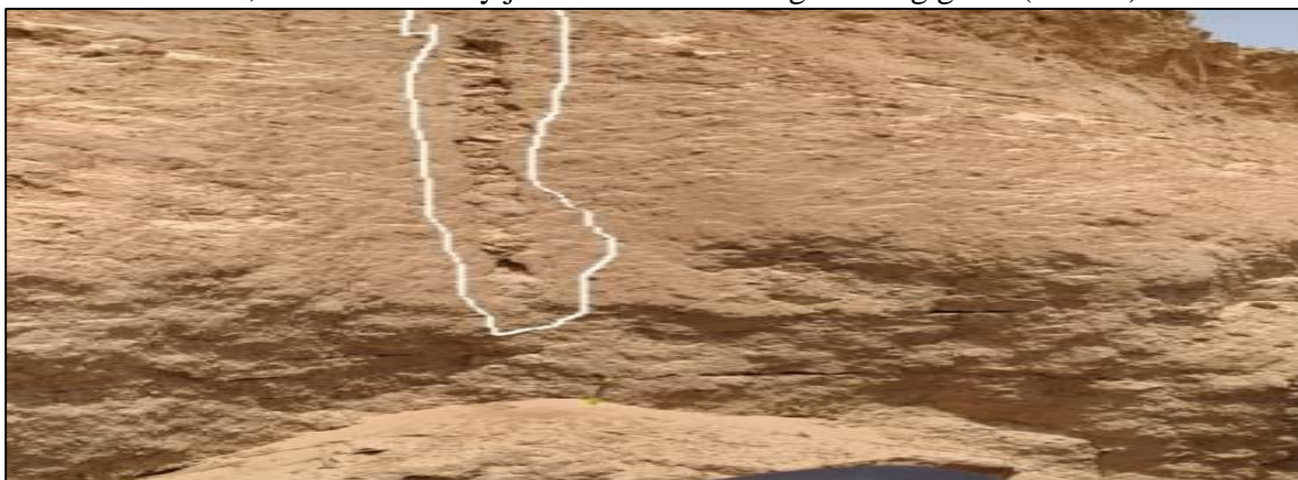
Plate 2. Claystone deposit with infilling grout joint
